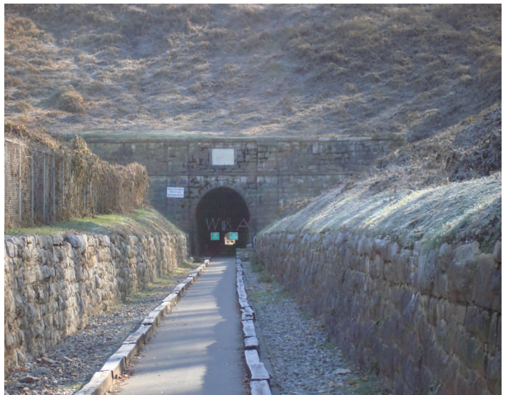
The Western & Atlantic Railroad tunnel at Tunnel Hill
